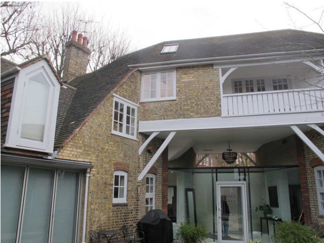
EAST SIDE COURTYARD
