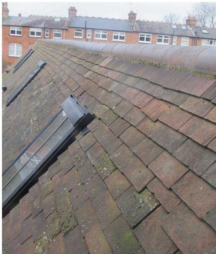
EXISTING ROOF TILES
