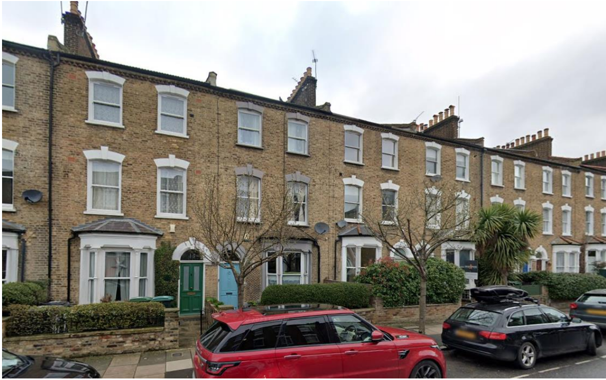
Figure 2: Street view image showing 16 Perth Road.
