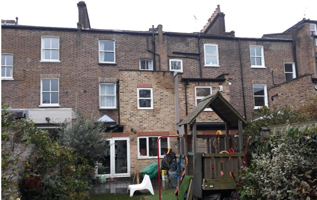
Figure 6: image showing the existing extension at properties 16 and 14 Perth road.
