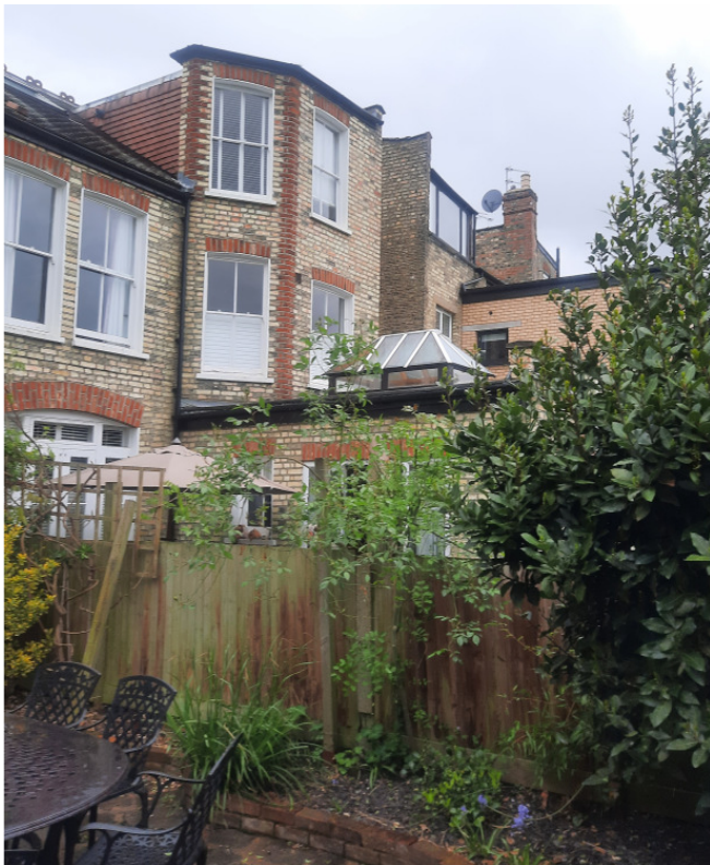
Rear garden view of existing extension at No.264
