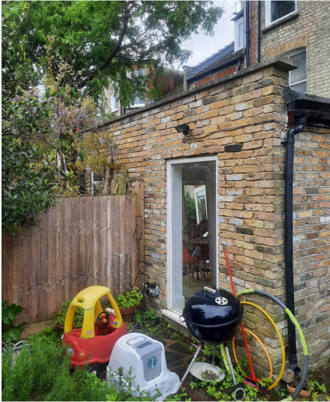
Rear garden view of existing extension at No.260
