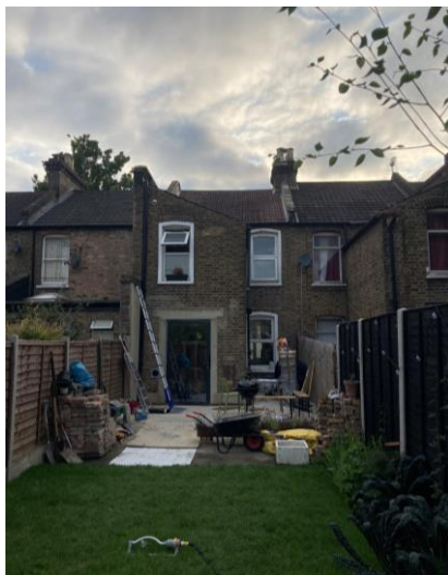
Photo of rear elevation as existing
