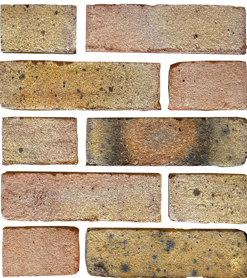
B Facing Brickwork Type 02 - Building A1, A2, C2, C3, D3
