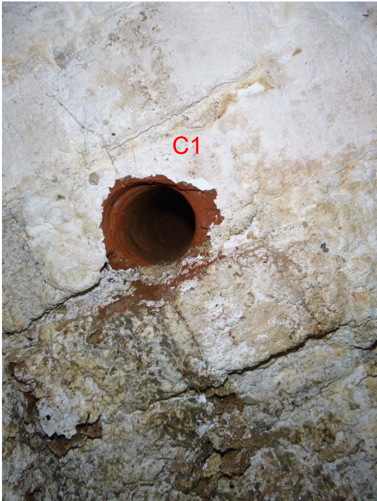
Photograph 11 Location C1 core hole.
