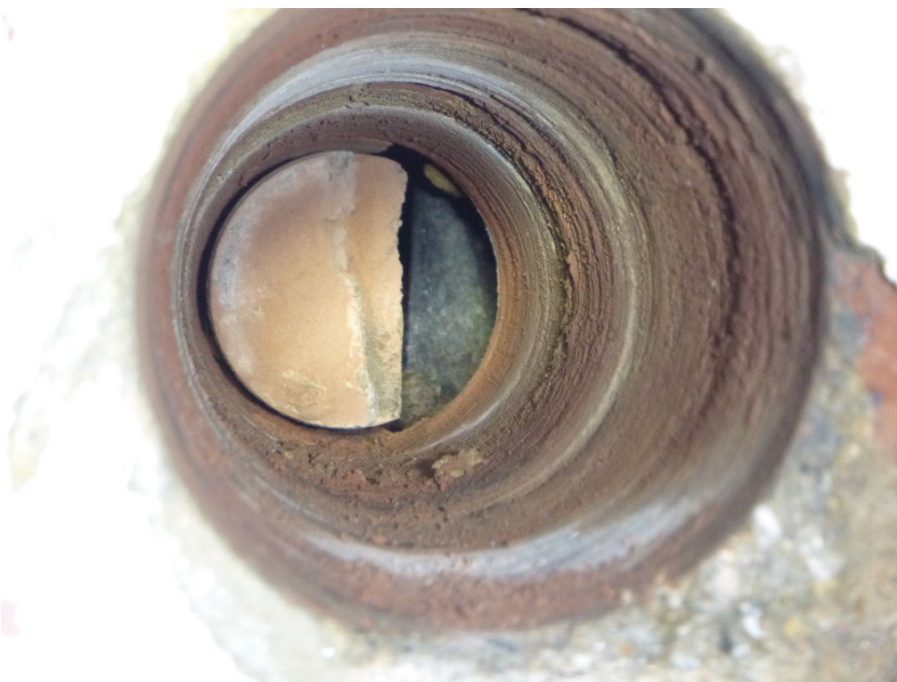
Photograph 5 Location A2. No apparent voids in brickwork. Manhole behind.
