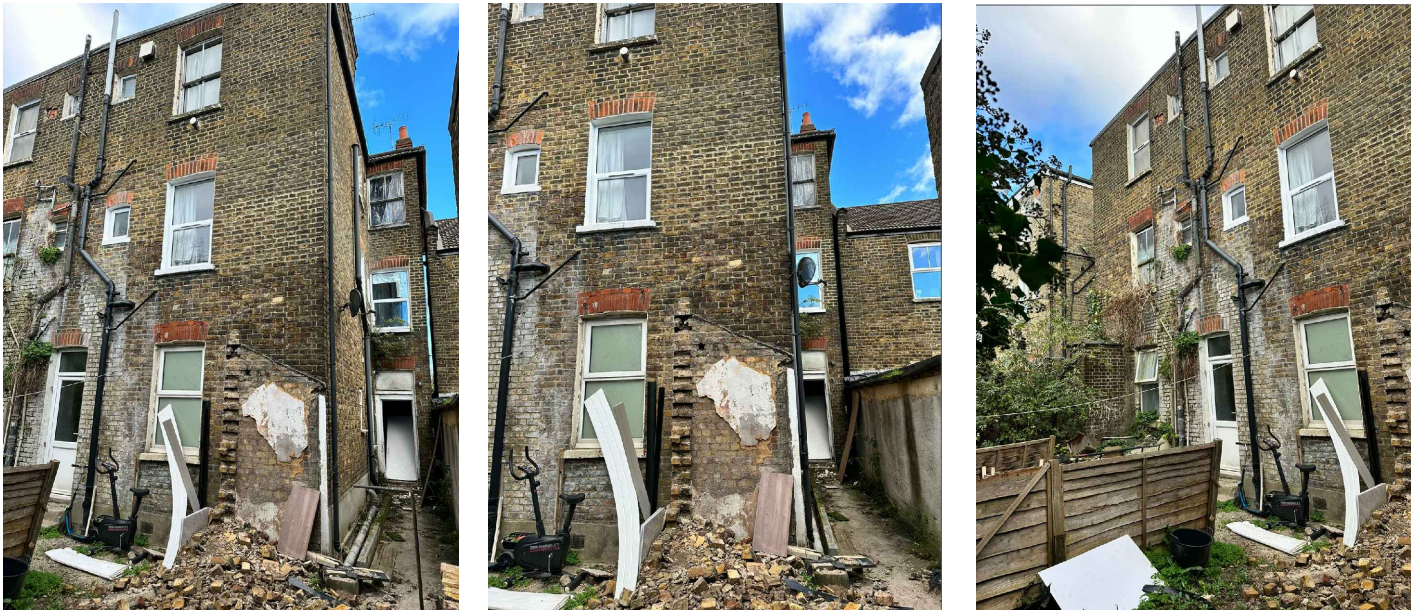
EXISTING REAR PHOTOS
