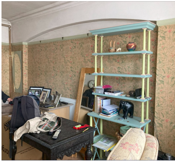
Room F prior to strip out
