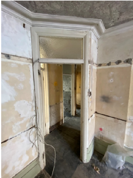
Oblique doorways with clear storey window integrated into door opening
