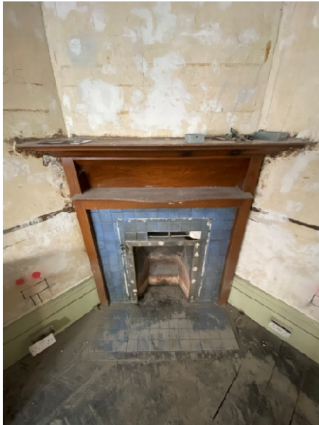
Room F fire place surround
