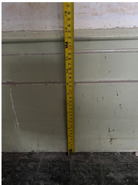
Skirting board detail with likely 220mm high add on
