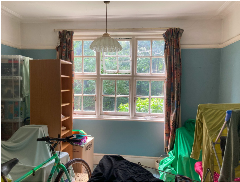
Room G prior to strip-out
