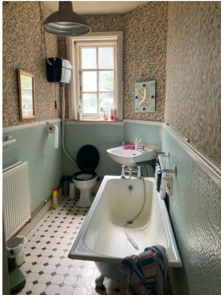
Room H prior to strip-out
