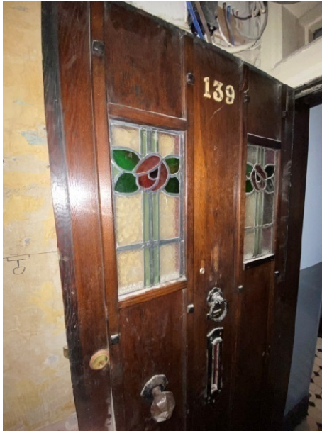
Original flat front door with lead framed glass
