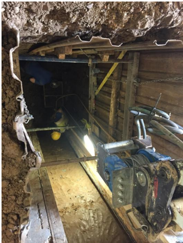
Shored Excavation for an underpin
