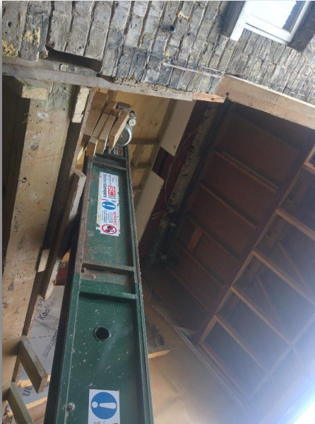
Conveyor to Remove Excavation Arisings
