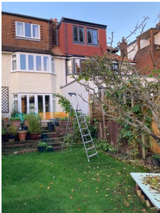
View of existing rear dormers to No 19 and No 17
