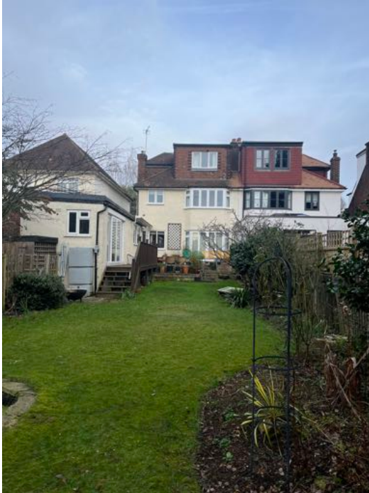
View of existing rear extensions to No 19 and 17
