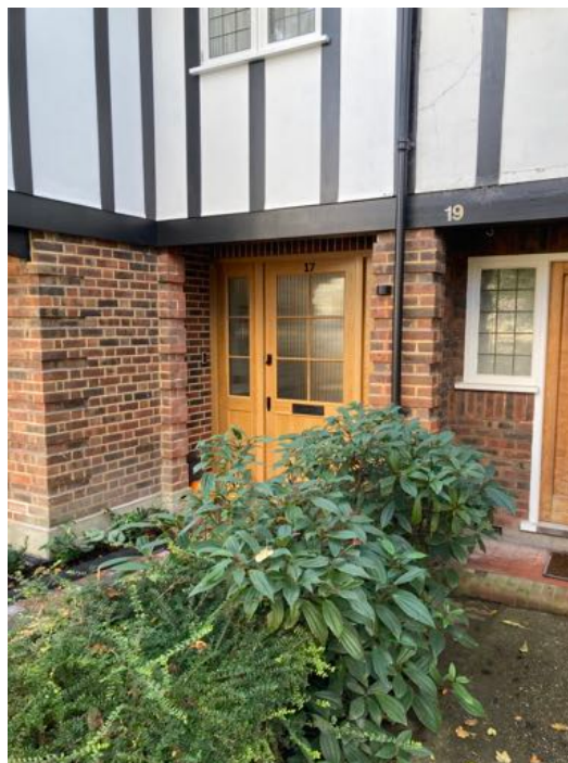
View of existing front doors to No 17 and No 19
