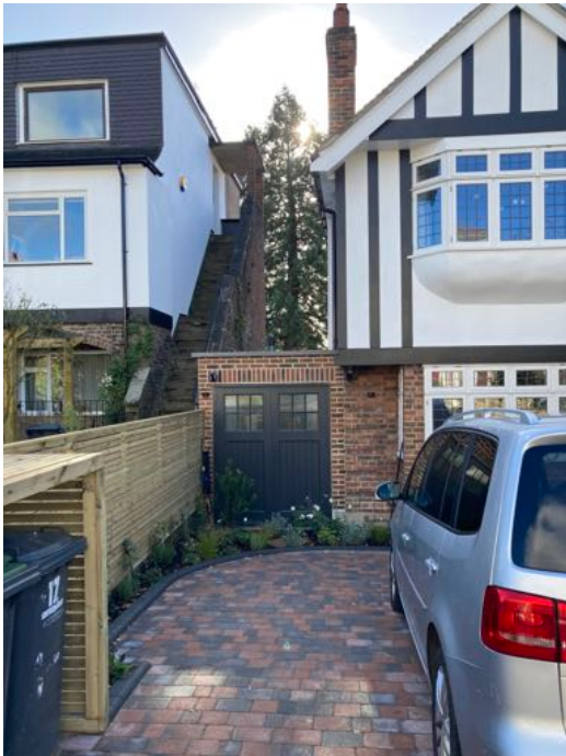
View of existing front extension to No 17
