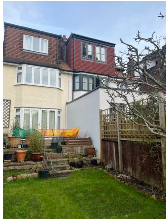
View of existing rear extension to No 17
