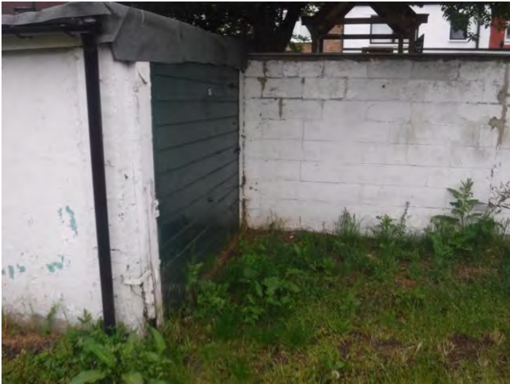
Door of one of the garages on the northern boundary.
