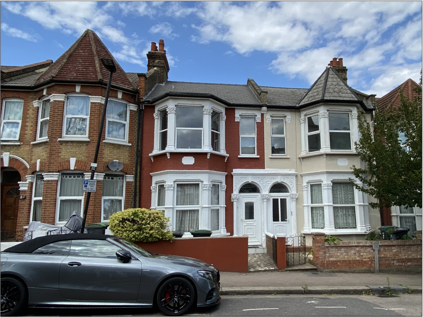
Existing front of property
