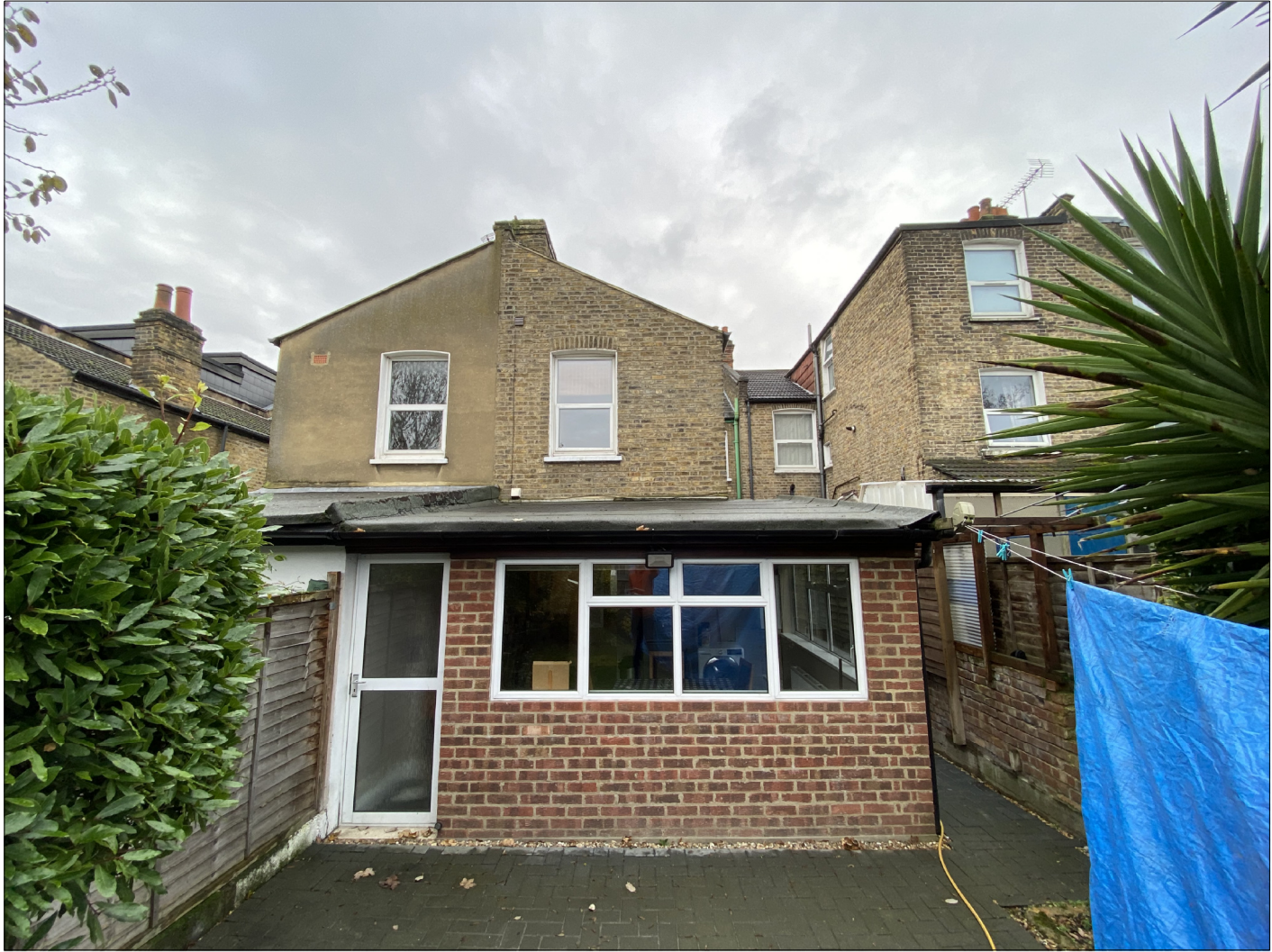
Existing rear of property
