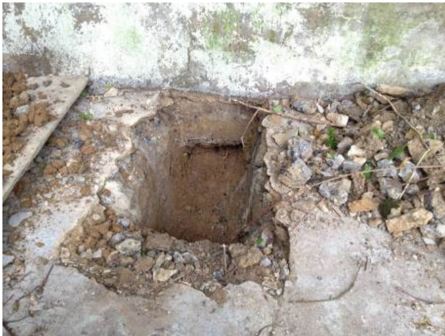
Figure 3 , hand pit dug at the Southern boundary wall.
