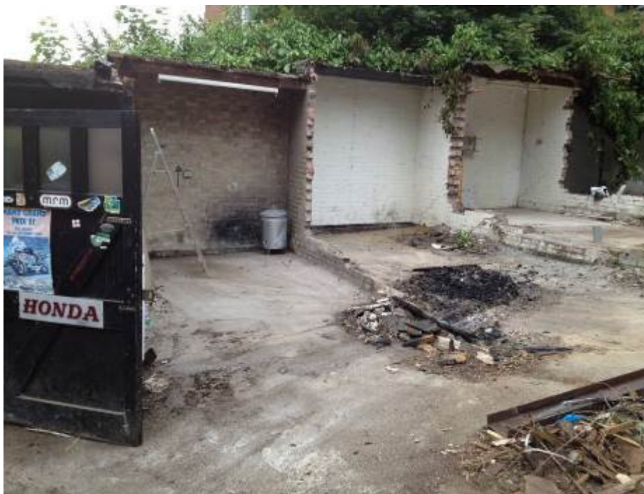
Figure 2 , Looking East towards the demolished garages.
