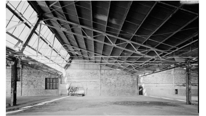
Figure 3.14 (Above): FORD Richmond Assembly Plant - View to east showing one of the openings in the second floor east wall through which a conveyor once passed for moving body panels to and from the second floor.
