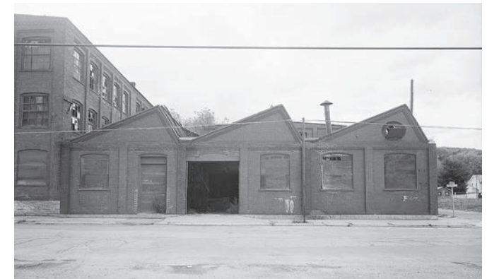
Figure 3.15 (Above): Front elevation of Building, showing closeup of sawtooth roof. - Merrill Silk Mill, 233 Canisteo Street, Hornell, Steuben County, NY Photos from Survey HAER NY-126.
