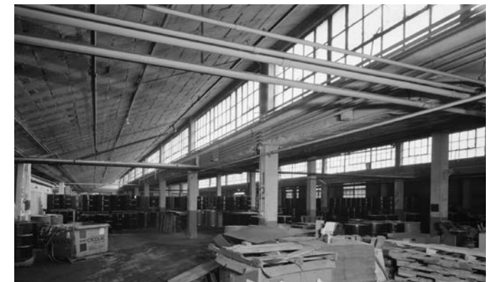
Figure 3.16 (Above): First floor, Steel Frame warehouse, sawtooth roof monitor, detail, looking north east, Buhl Sons Company complex, 120-234 Adair Street, Detroit, MI Photos from Survey HAER MI-13.
