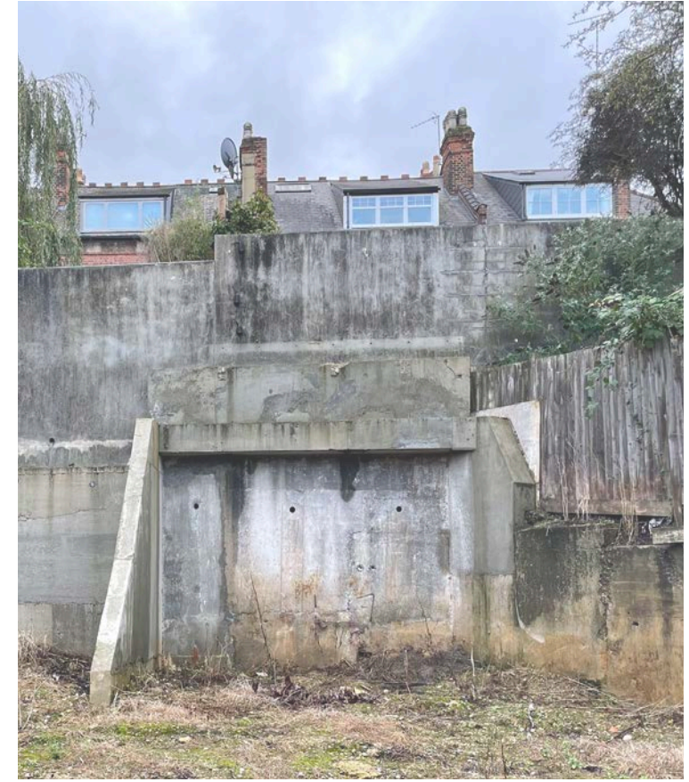
Photo 07: Existing buttress retaining Church Crescent garden wall.
