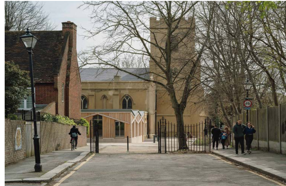
Figure 1.1: St Marys Walthamstow, restoration and cafe' extension.
