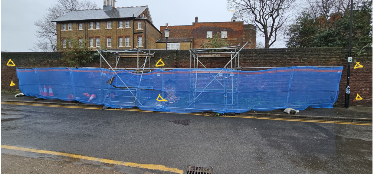
View Showing Scaffold Erected (by others) and Proposed Movement monitoring targets
