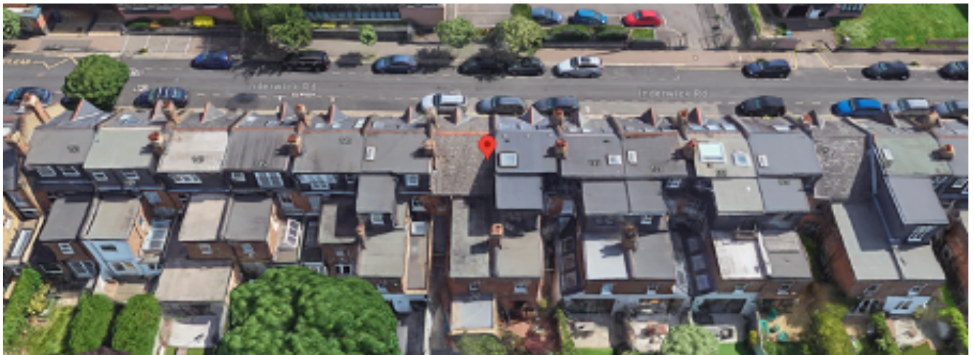
Rear Terrace Setting of 125 to 151 Inderwick Road
