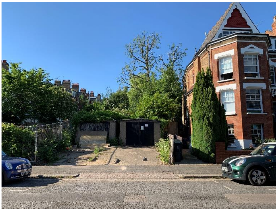
Fig.9 the site viewed from Church Crescent
