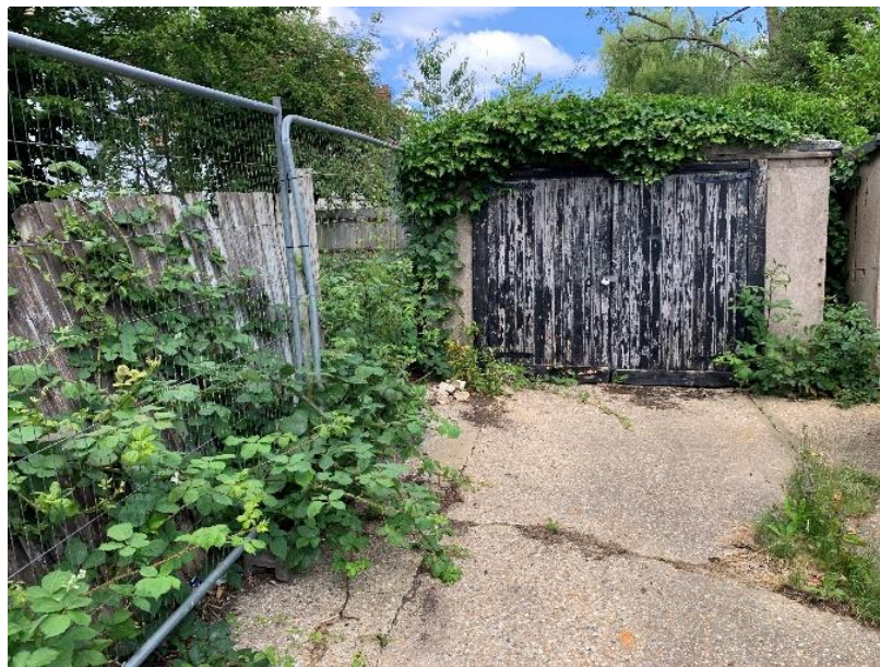
Fig.11 Detail of the western boundary fence
