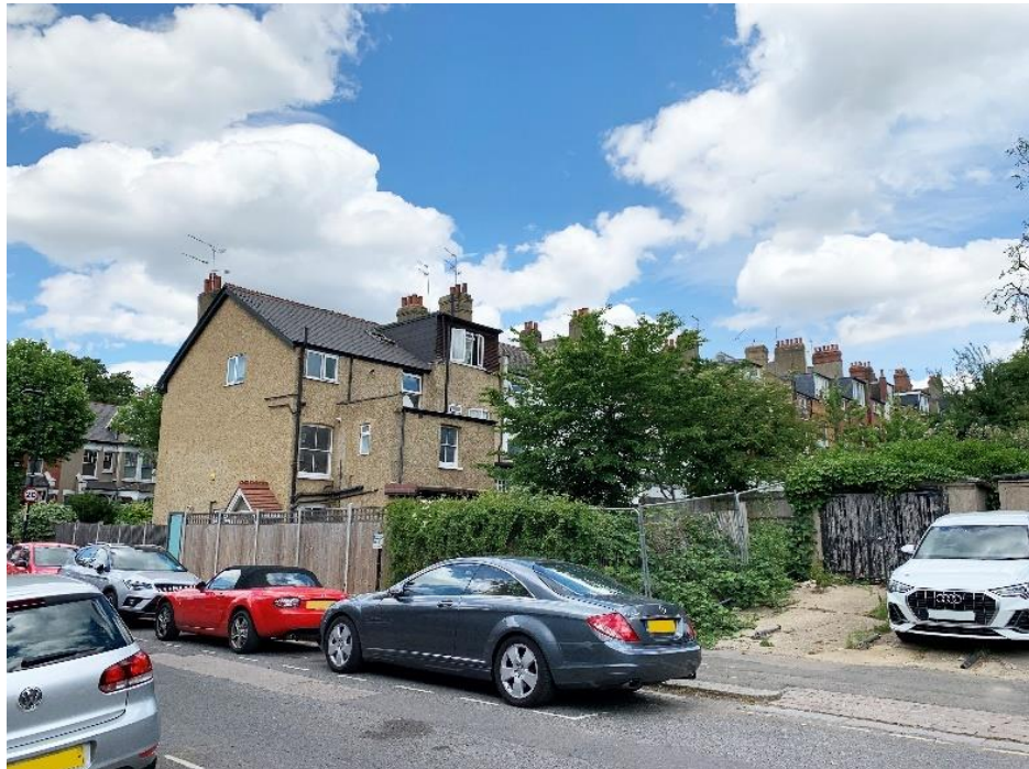
Fig.14 Location of the back end of the 168 Muswell Hill Road building
