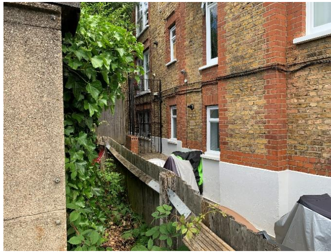
Fig.10 Detail of the eastern boundary fence
