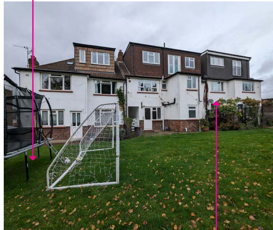
View from communal space at rear
