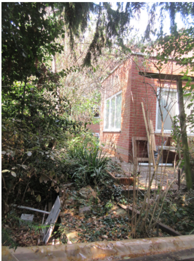
Rear of #69 site - taken on 17/8/22
