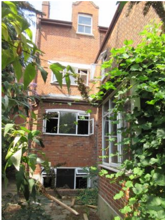
Rear of #69 site - taken on 17/8/22
