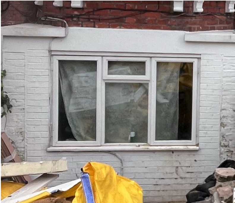
Photo of existing single glazed timber casement windows.
