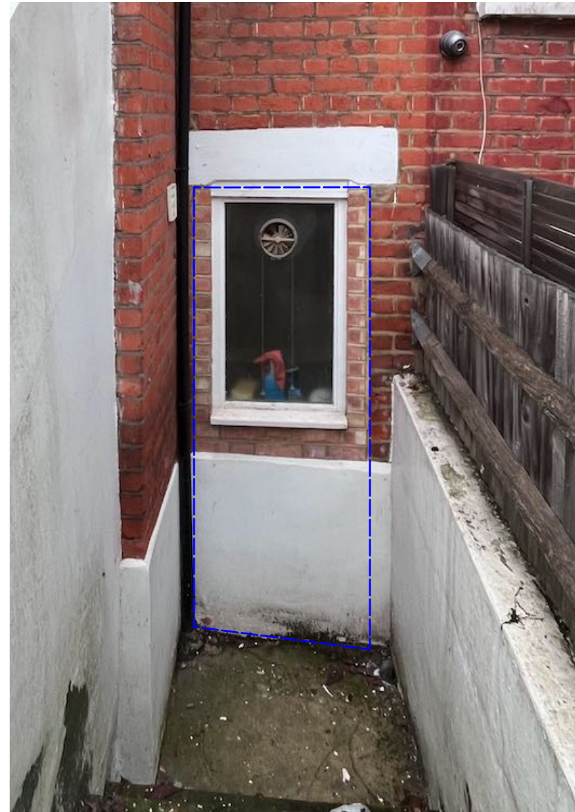
Photo of existing window at basement level.
