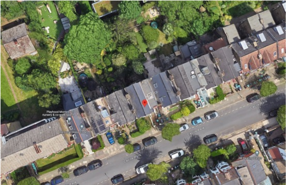
View to rear of house
