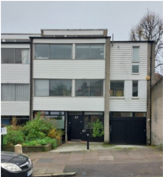
EXISTING FRONT ELEVATION (Main House) - PHOTO NTS
