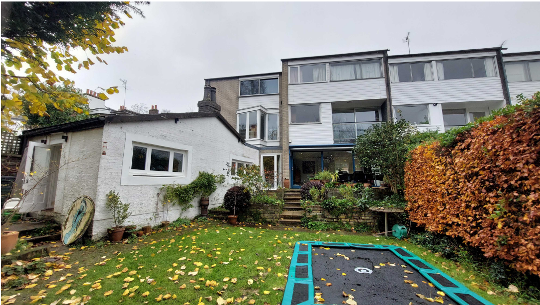
EXISTING REAR ELEVATION (Main House) - PHOTO NTS
