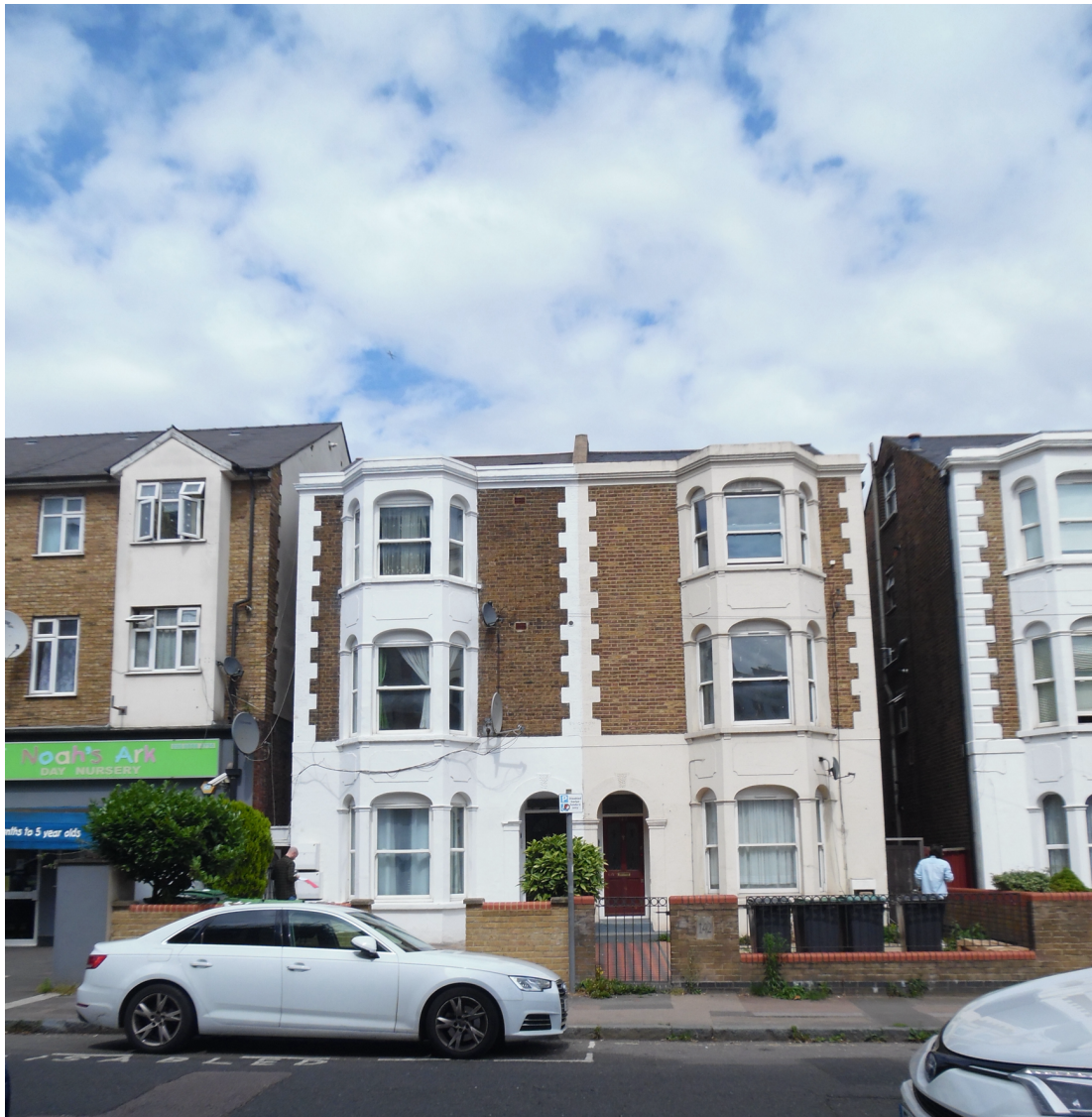
Front view from Mayes Road
