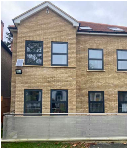
Local example of properties with front lightwell 35, Maidstone Lane
