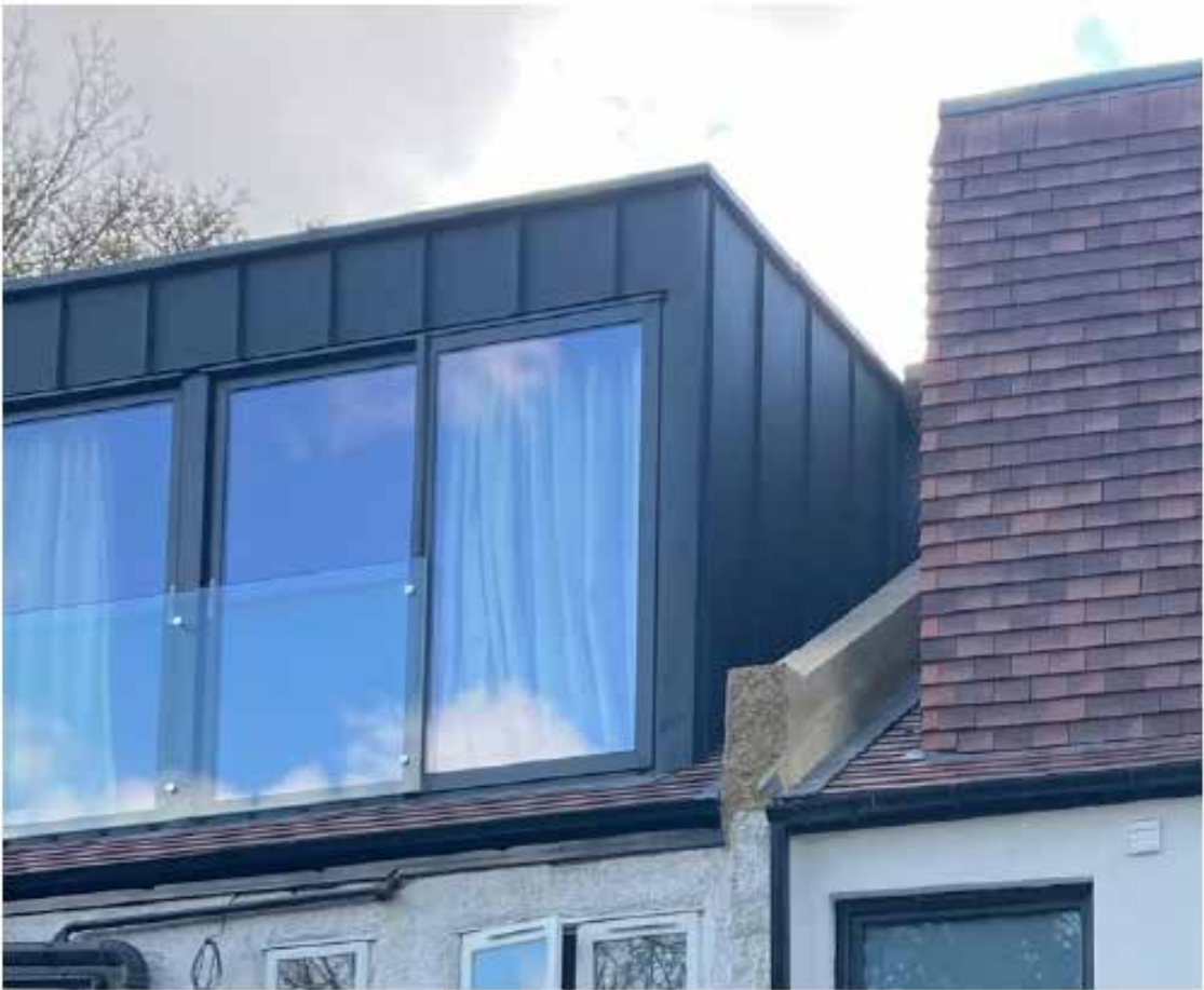
#86 Priory Gardens Rear Dormer Extension
