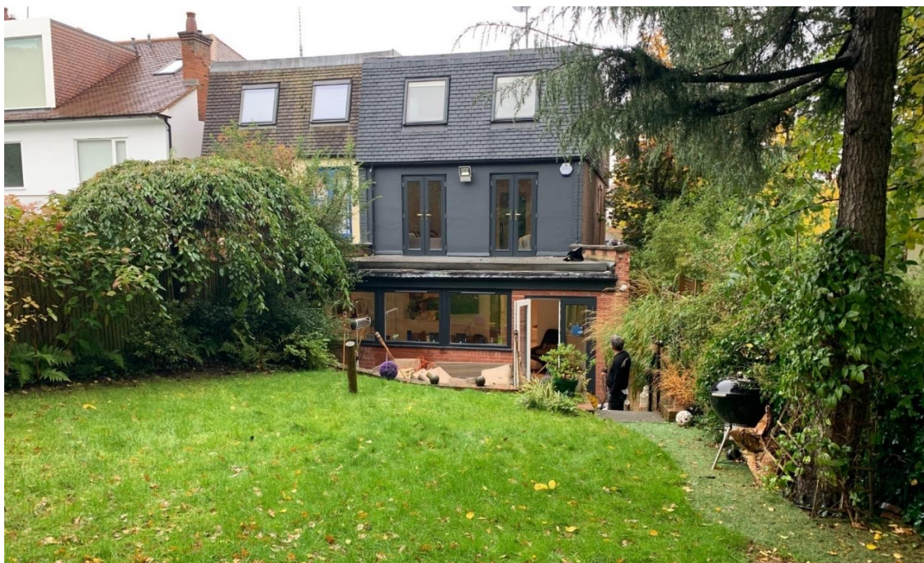
Existing Building - Rear Elevation
