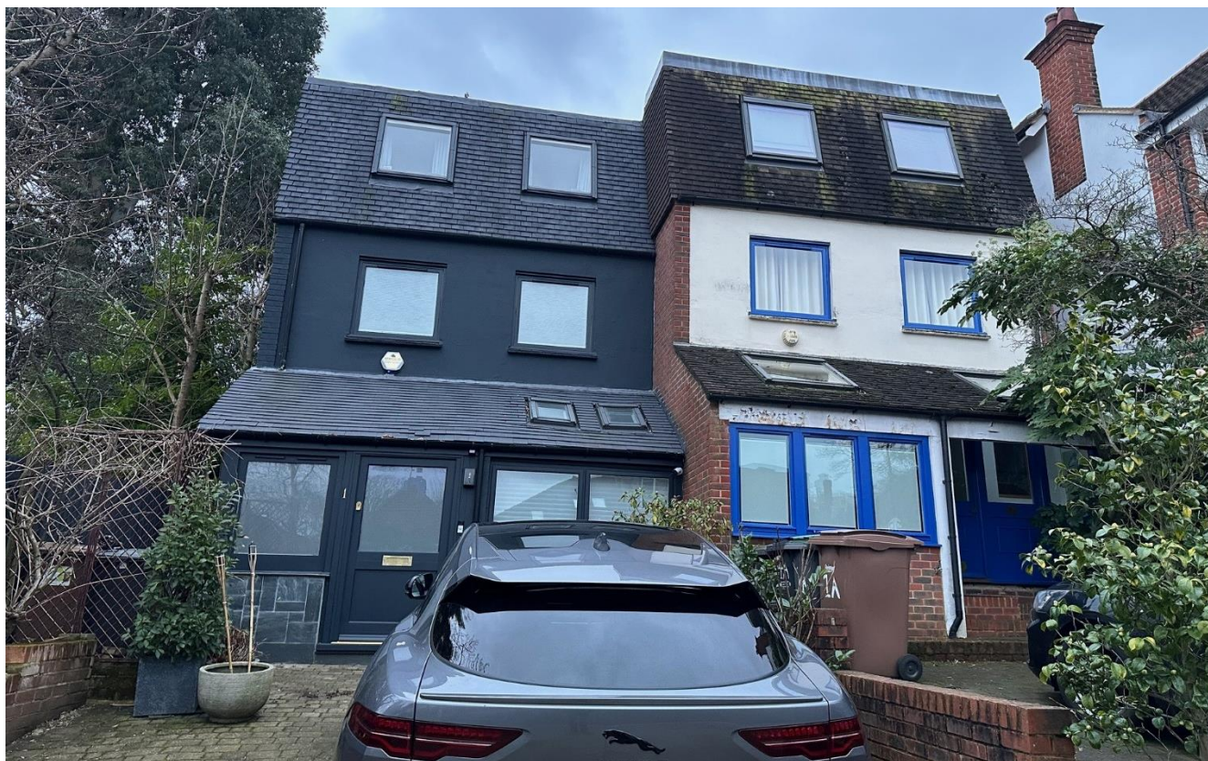
Existing Building - Front Elevation
