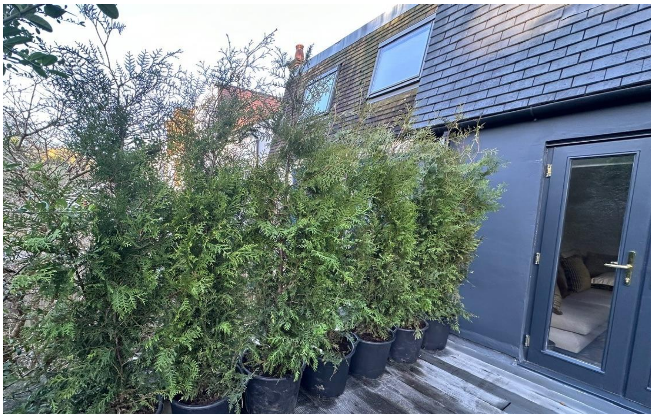
Existing Building – Existing Rear Extension (looking towards the neighbour)
