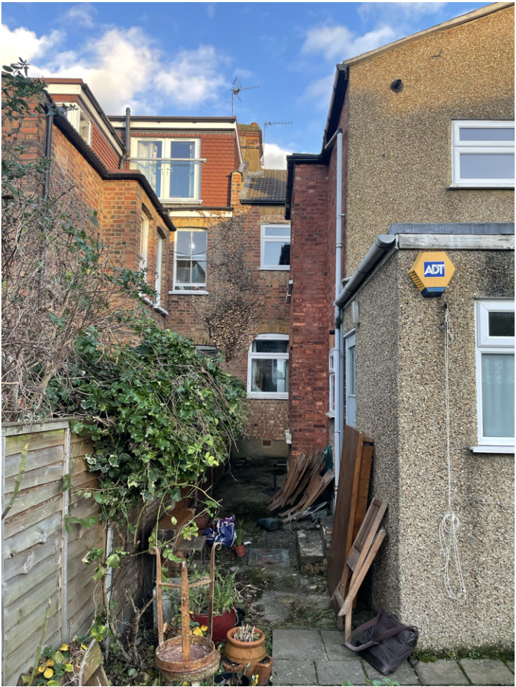
Above: Photo showing the space between the outriggers to No. 13 and No. 15
