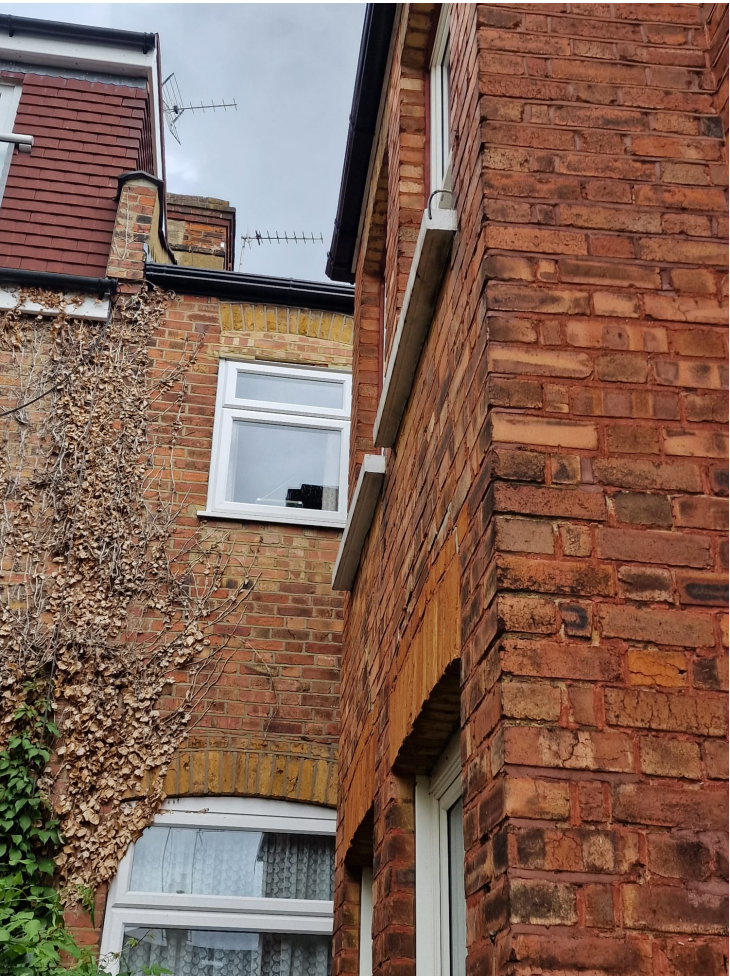
Above: Photo of the existing party wall condition with the loft conversion to No. 17. This photo also indicates the infilling of the existing window opening to accommodate a smaller UPVC window
