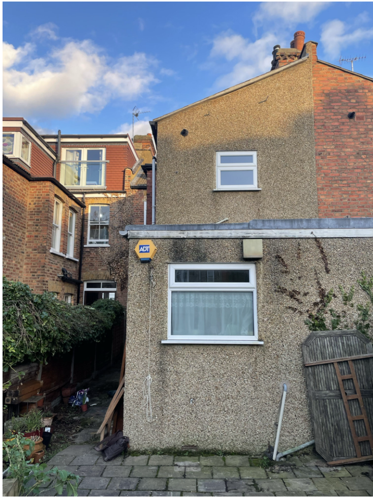
Above: Photo of the rear elevation, showing the rear dormer and outrigger extension to No. 17 Princes Avenue. It also shows the existing pebble dash render to the rear elevation.
