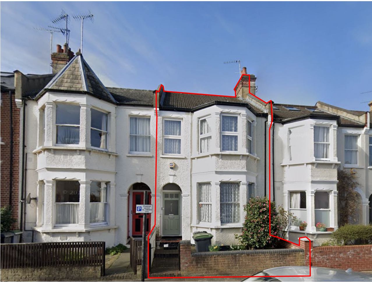
Above: Photo from Princes Avenue of the site (site highlighted in red) No. 17 is to the right hand side, with the three rooflights facing the road and the ridge having been raised to accommodate a loft conversion
