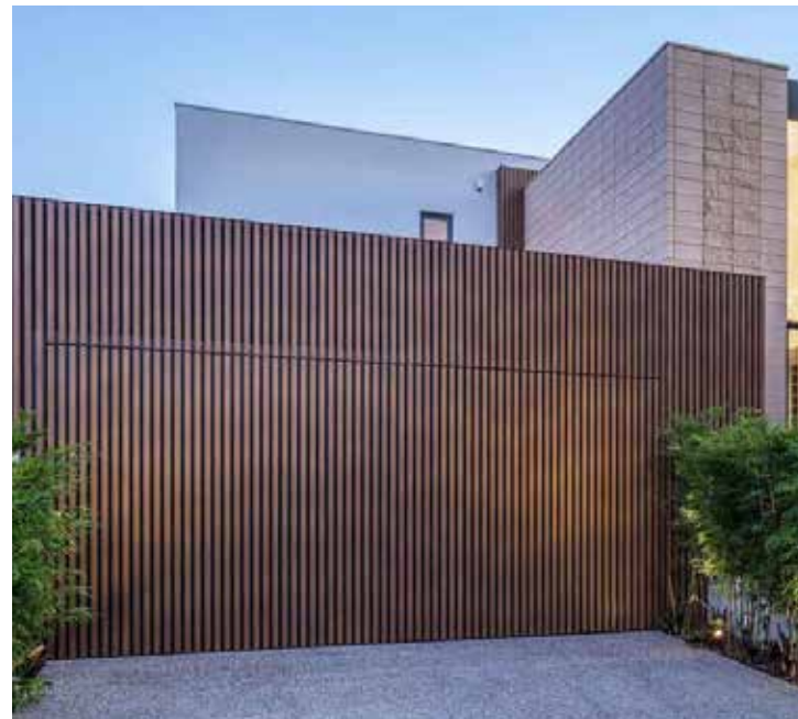
Timber effect batten cladding
