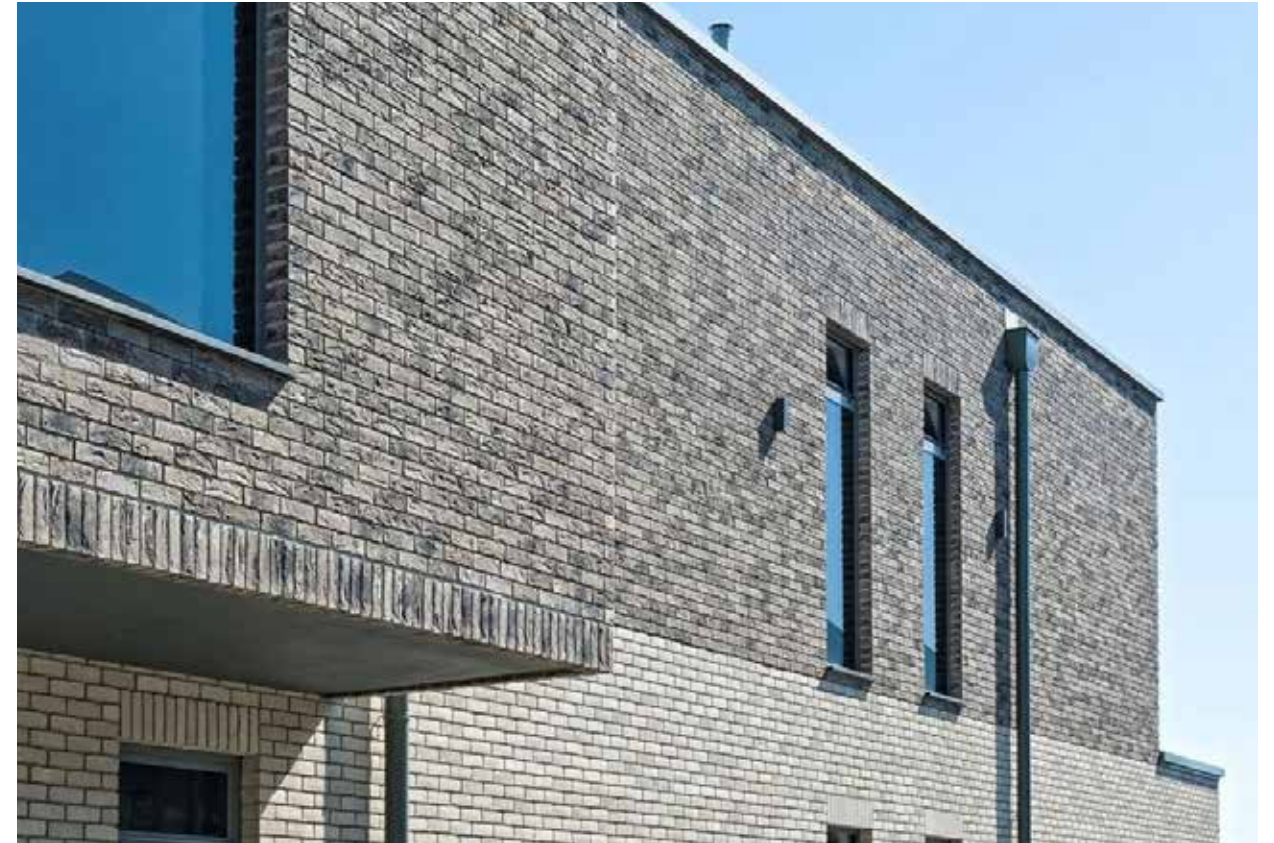
Brickwork - utilised with contemporary detailing
