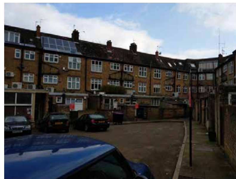
M | View looking at properties at the end of Aylmer Parade
