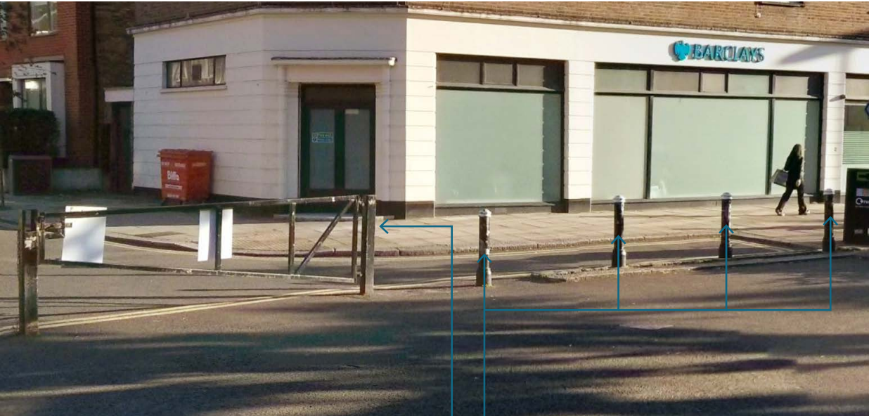
Existing Gate - to be replaced with new gate as approved scheme and detailed in condition 4 submission
