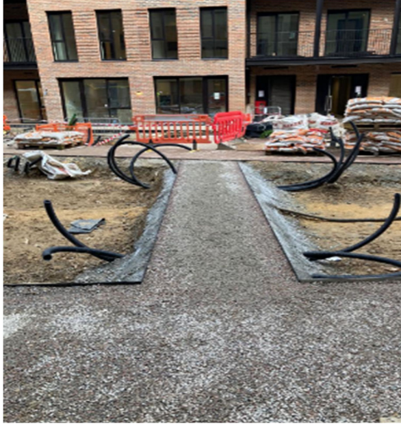
Photo 3: Image of the courtyard during construction with hardstanding and dug out areas for soft landscaping (Client Provided Image).
