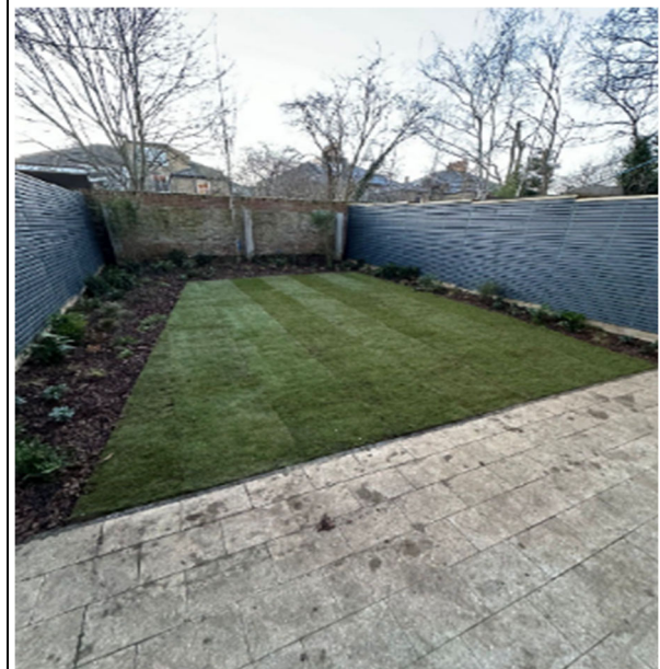
Photo 4: A photo of the garden areas following installation of turf and fencing following EPS' visit (client provided image).
