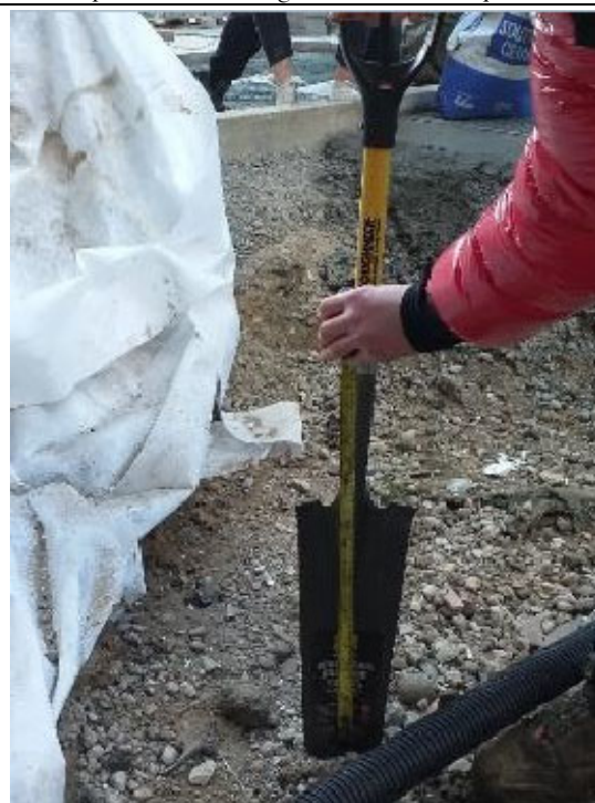
Photo 8: Photo showing the depth of cover to be installed in the final soft landscaping area with the membrane that separates the made ground from the topsoil.
