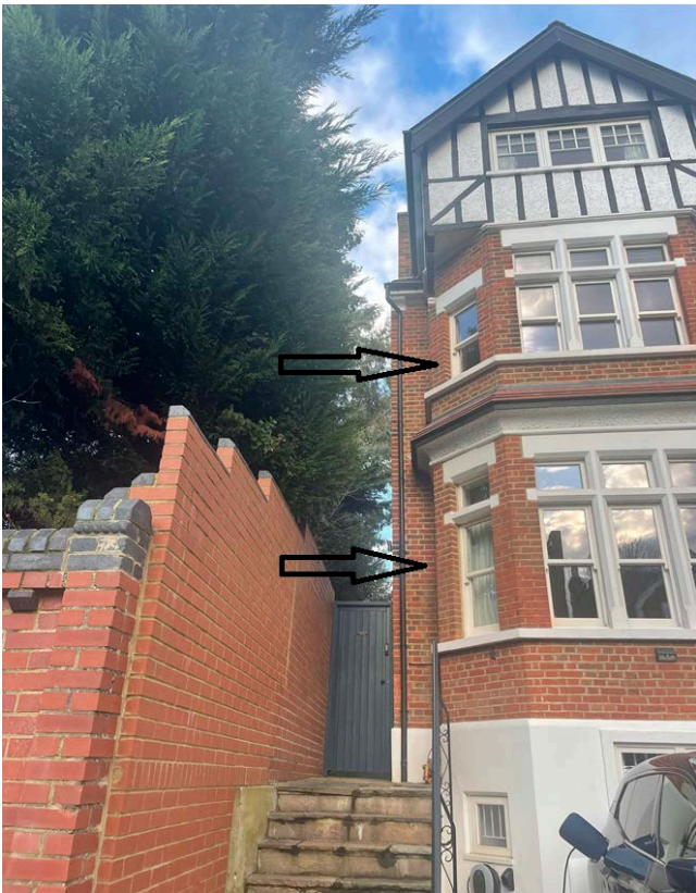
Picture Six – Living room and bedroom windows at 45 Clifton Road which the windows of the new dwelling will look directly into.
