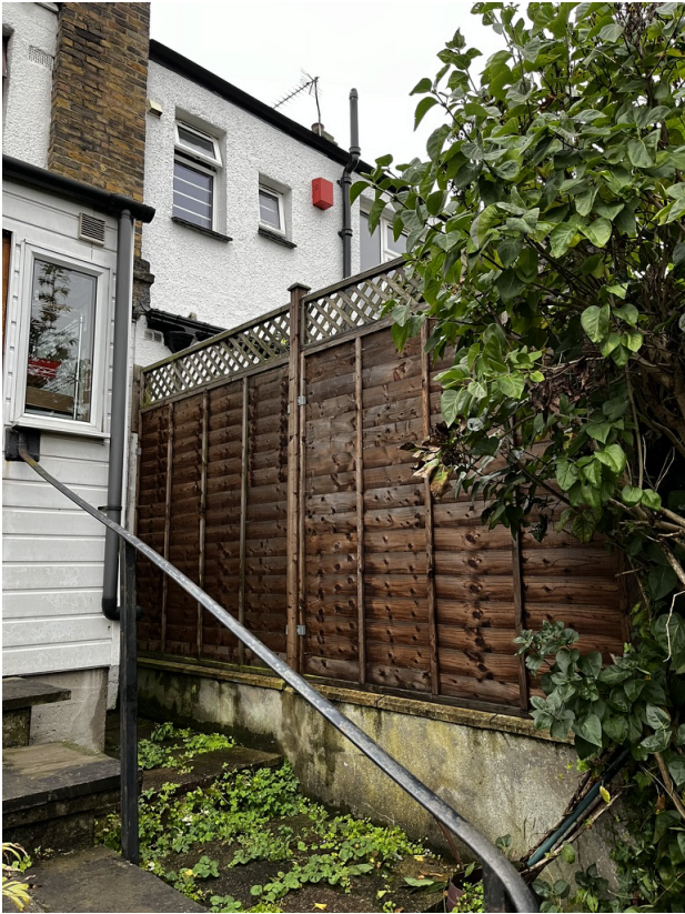
High fence to boundary of 99 Higham Road
