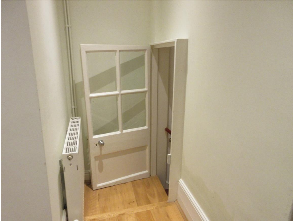
Figure 84: Hallway (i.e. G2 in Figure 36), with historic door to basement, shaved off at the bottom.
