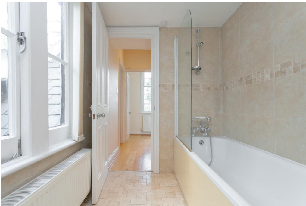
Figure 71: Bathroom/corridor (i.e. F1 in Figure 36). Note modern casements on left. (Source: Stonebridge & Co.)
