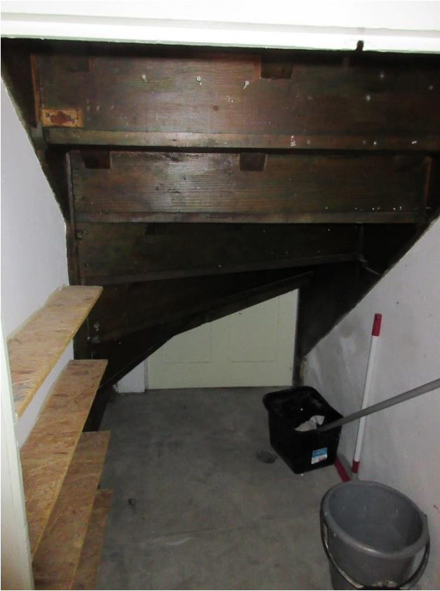
Figure 57 (left): Area beneath north staircase. The timber to the underside of the treads may well be historic.
