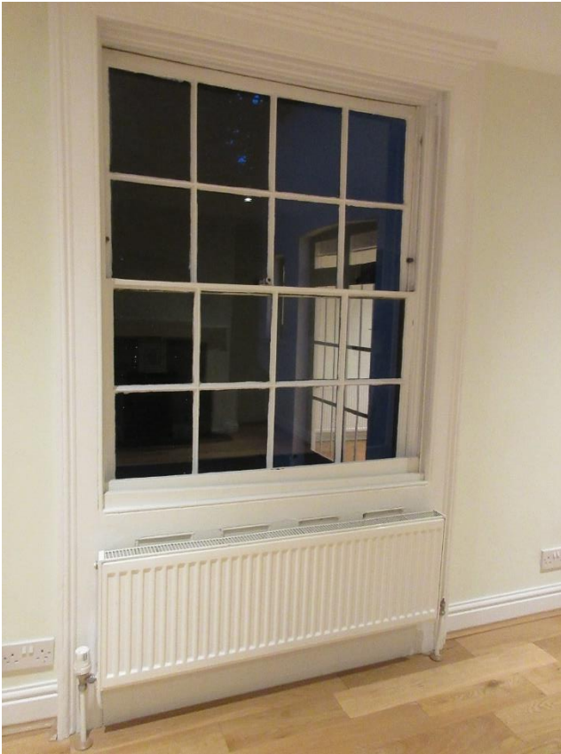
Figure 65 (left): Dining room (i.e. G4 in Figure 36). Note historic sash window, with vertical built-in sliding shutter.
