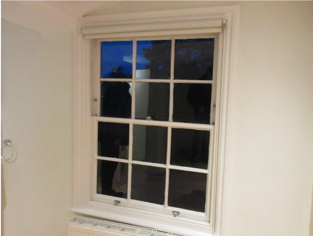
Figure 81: Bedroom (i.e. S1 in Figure 36). Note historic sash window.
