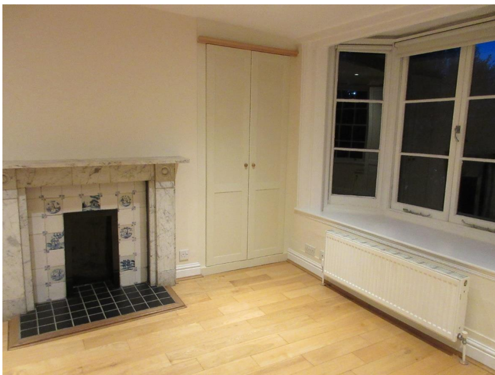
Figure 69: Bedroom (i.e. F3 in Figure 36). Note fireplace which is likely a reproduction, modern built-in joinery and modern casement windows.
