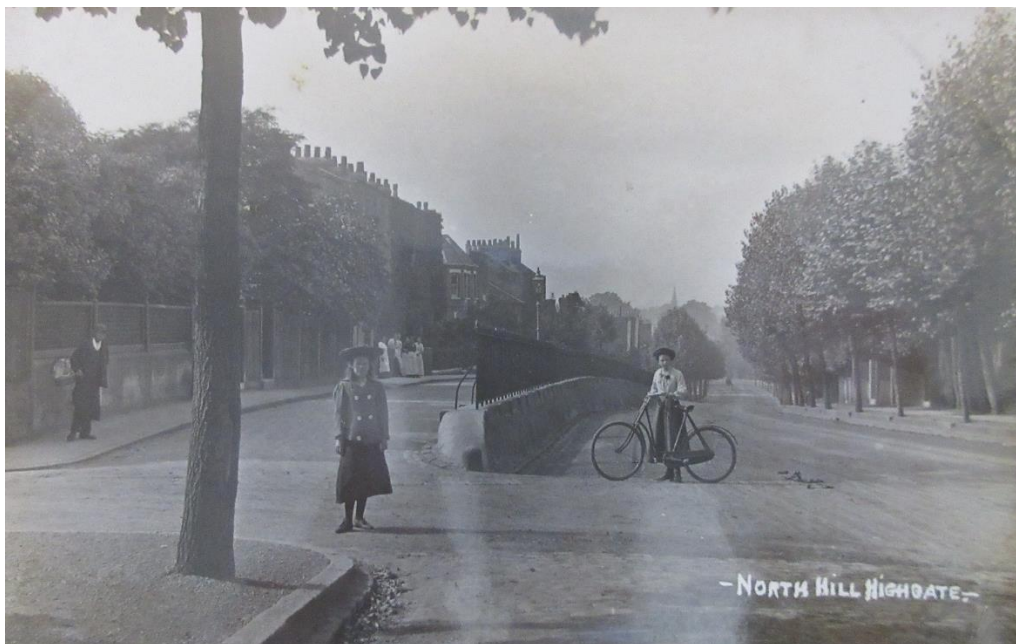
Figure 25: 1910 postcard of North Hill, looking northward from the junction with View Road and Church Road. Subject site is to the right, hidden behind trees. (Compare with Figure 3.)
