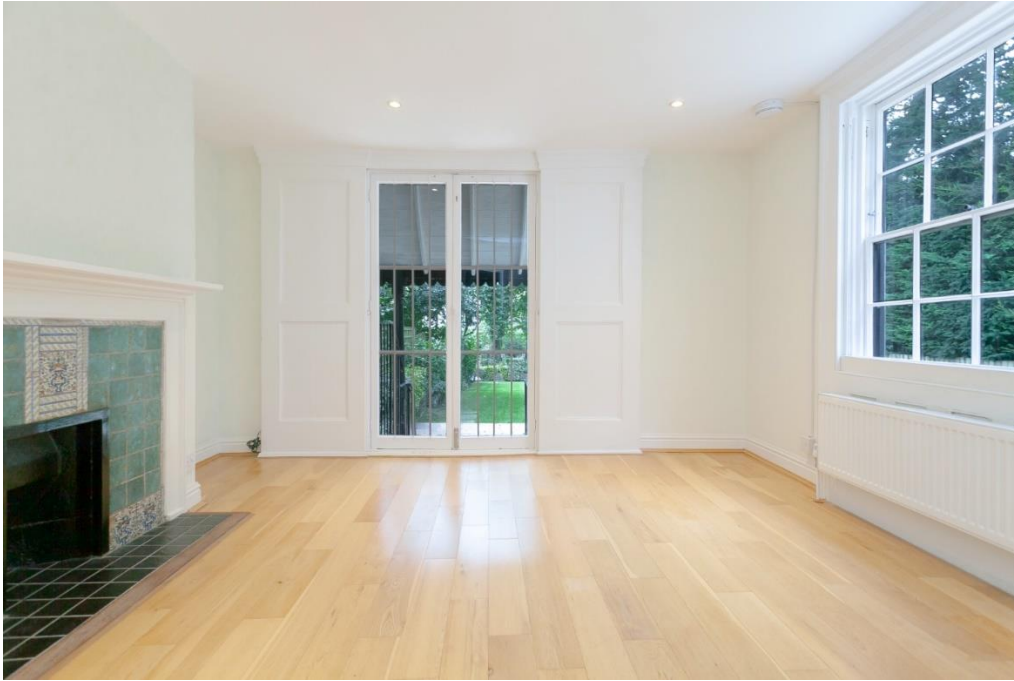
Figure 63: Dining room (i.e. G4 in Figure 36). Note fire surround with tiling which may be historic, modern skirting, modern fenestration and modern downlighting. (Source: Stonebridge & Co.)
