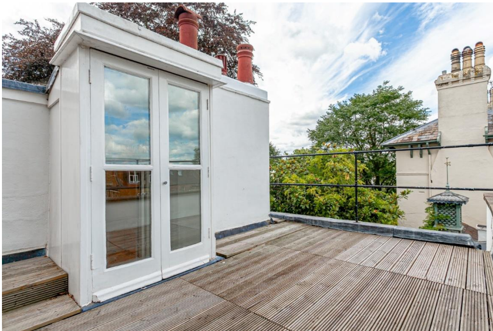
Figure 35: Roof terrace (accessed from second floor bedroom – i.e. S2 in Figure 36). (Source: Stonebridge & Co.)
