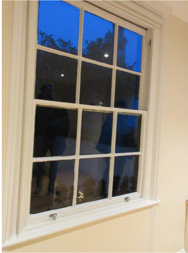
Figure 70: Bedroom (i.e. F3 in Figure 36). Note historic sash window.
