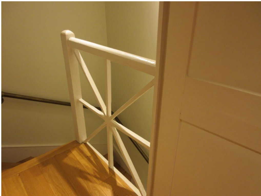
Figure 56: Historic balustrading by south staircase.
