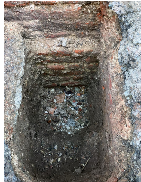
Trial pit for investigation carried out August 2023. Area of investigation indicated below.
