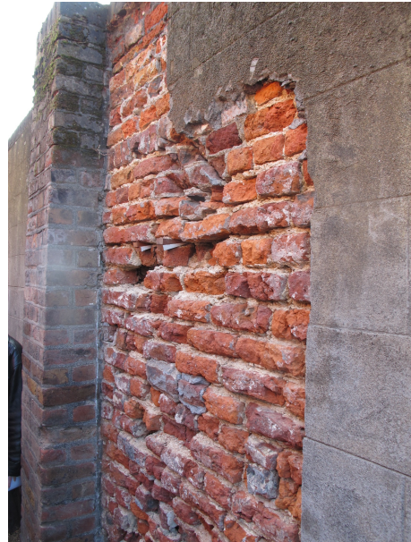
Render removal investigation (August 2023) in area indicated below.
