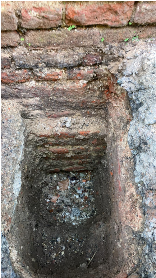
Fig 4: Photos of the trial pit investigation, August 2023
