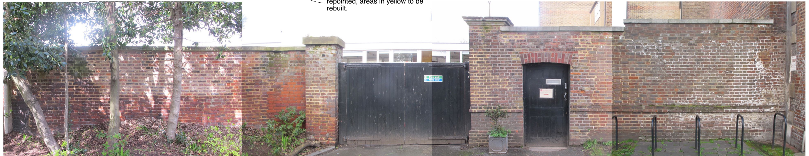
EXISTING PHOTO COLLAGE OF WALL
