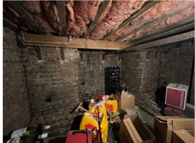
Fig.5: Existing cellar - front elevation with corbelled footings exposed
