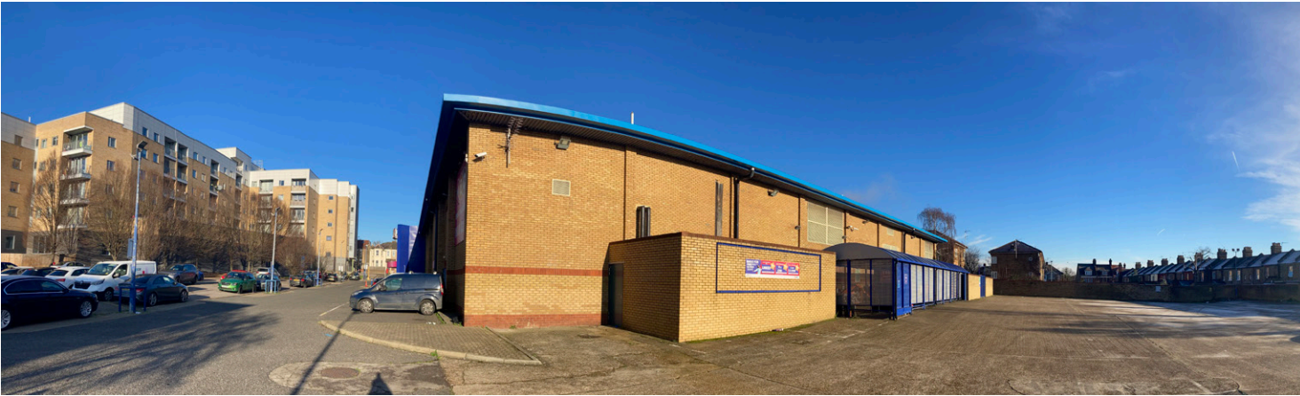
Figure 5.1: Panorama taken looking north-west from the south western corner of the existing building.
