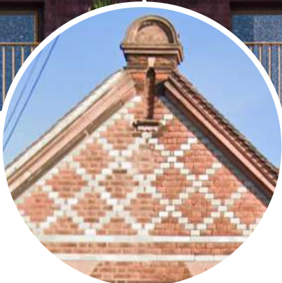
Pitched roofs and ornamentation
