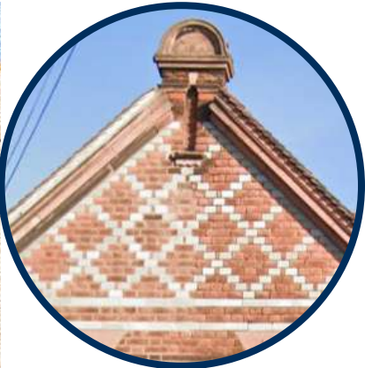
Pitched roofs and ornamentation
