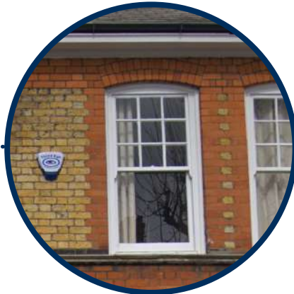
Brick windows surrounds expressed in change in tone
