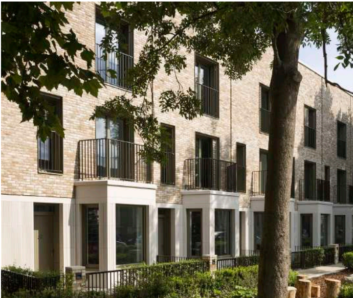
Futurehomes, Passivhaus, London
