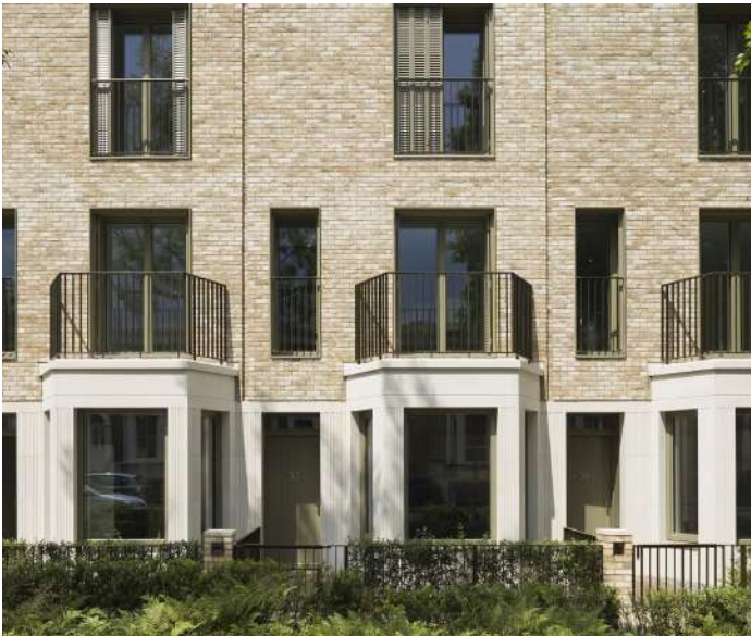
Futurehomes, Passivhaus, London
