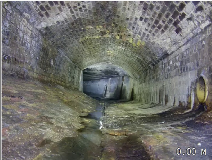
Start node type, manhole, reference MH19a
