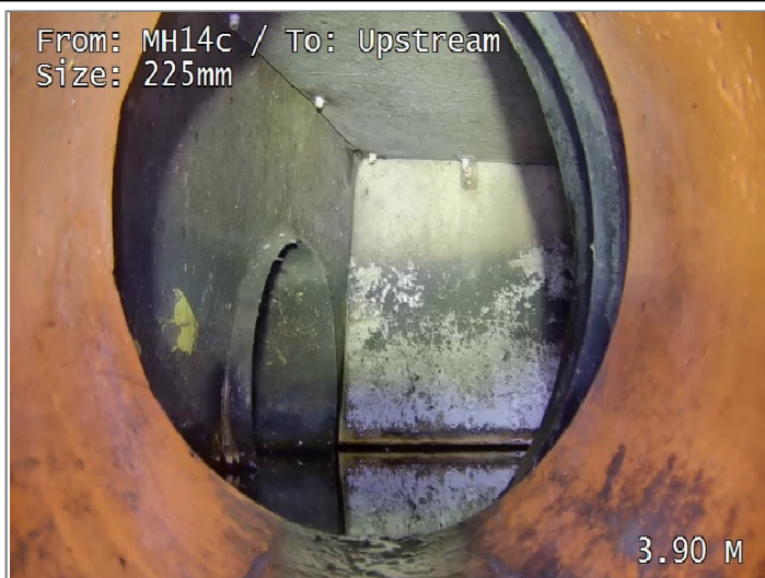
Finish node type, manhole, reference MH13
