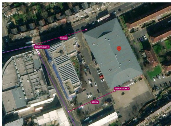
Figure 3.3 – Future Closest District Heat Network Connection Point. (circa 67 metres away)
