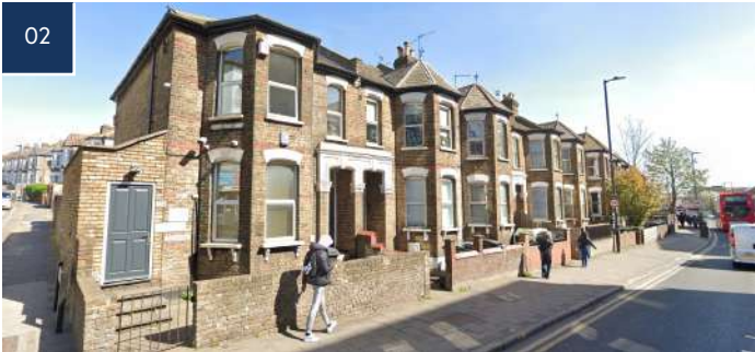
Terrace Housing (2 Storeys) Existing residential properties along Lordship Lane, Victorian/Edwardian 1840 -1910s
