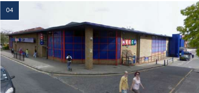
Mecca Bingo (2 Storeys) (Site Location)
