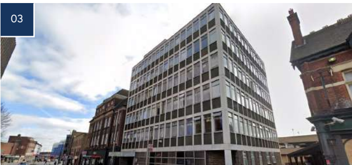
Greenwood House (6 Storeys) Residential building comprising of 1/2/3 bedroom flats.
