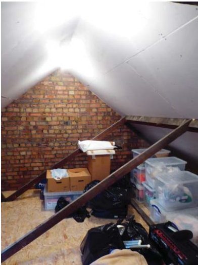
Loft space looking south
