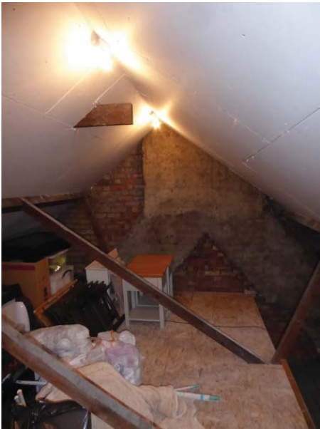
Loft space looking north
