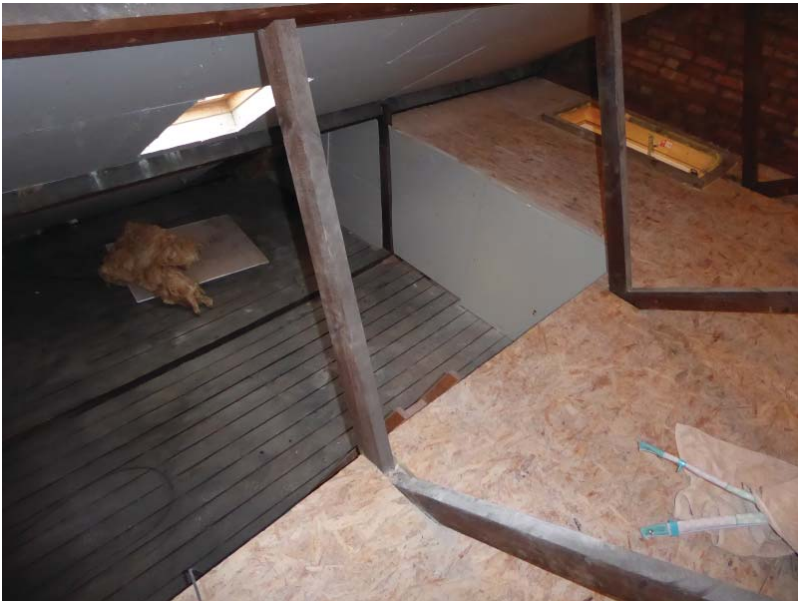
Loft space looking south-east
