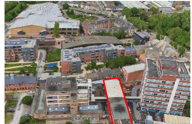
Four-storey development at rear of listed Town Hall with Bernie Grant Arts Centre beyond and Tottenham College and application site in red in foreground.(Google Earth)
