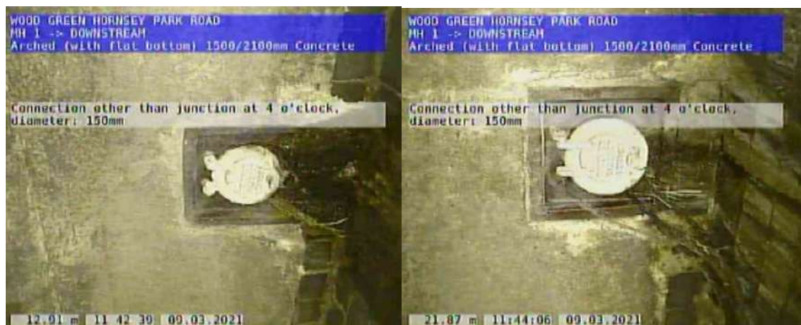
Figure 13 – Connections Found in Culvert Survey
