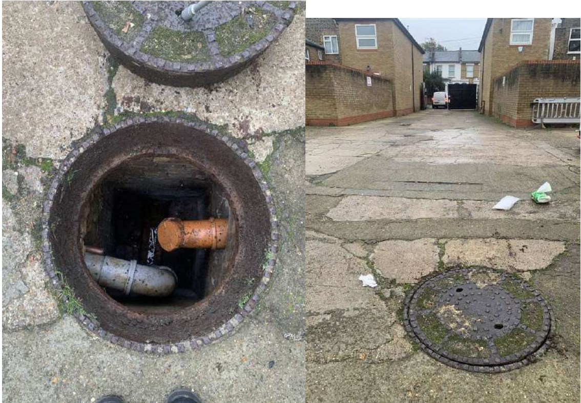
Figure 12 – Photo of Drainage Manhole from Site Visit
