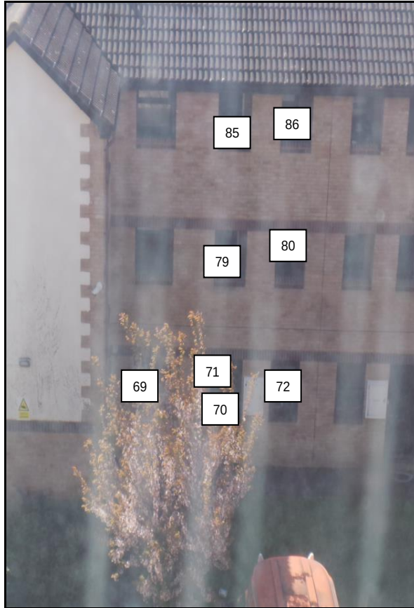
157 to 211 Portland Road
