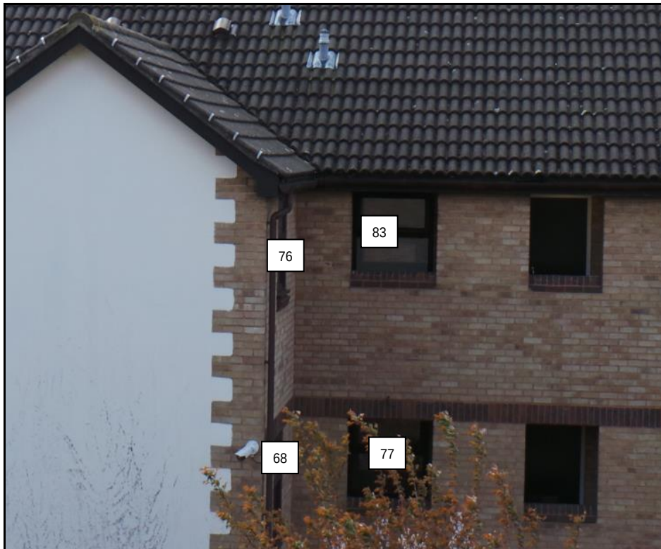
157 to 211 Portland Road
