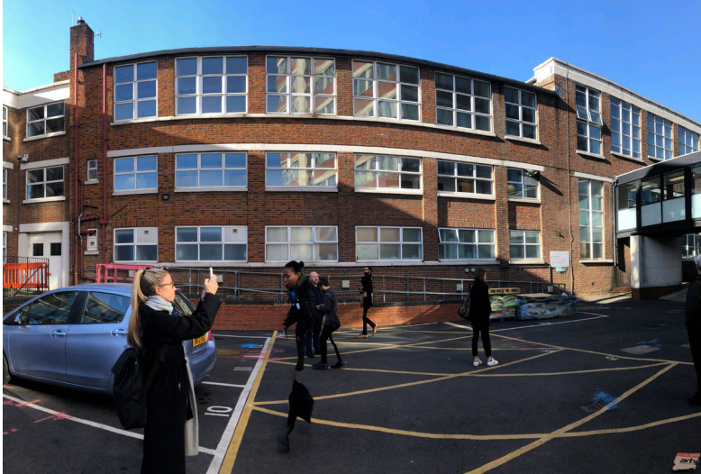
06. Existing Building to be demolished and link
