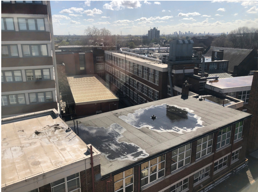
Site photos of existing building to be demolished
