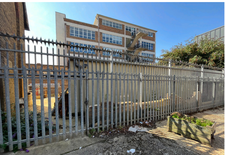
11. View from Isobel Place into the Site
