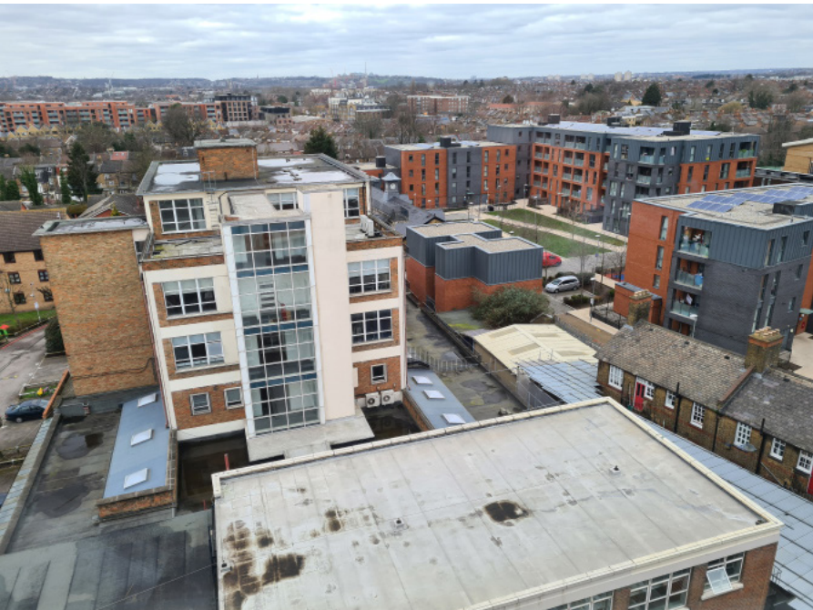
View of Building Block from Tower
