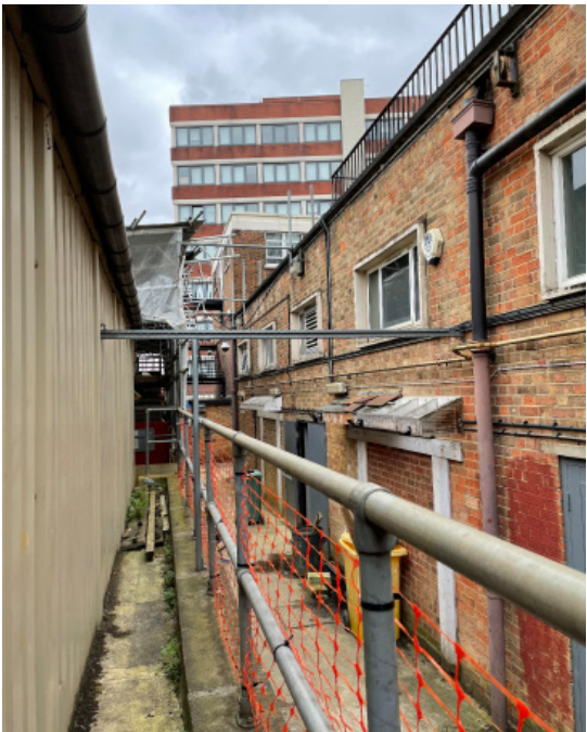
Perimeter of Building Block
