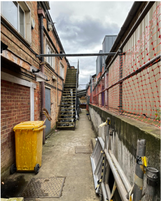
Perimeter of Building Block
